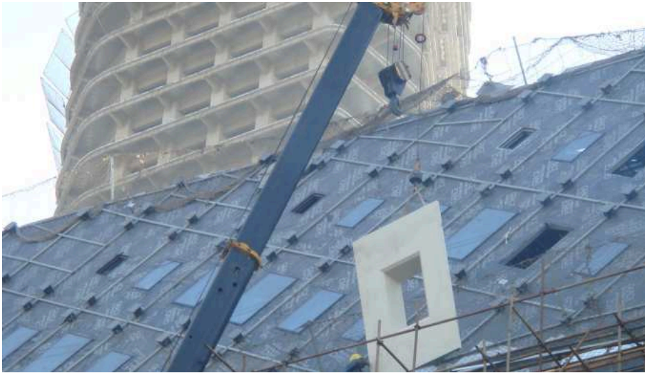
Figure 15 Panel installation on roof
