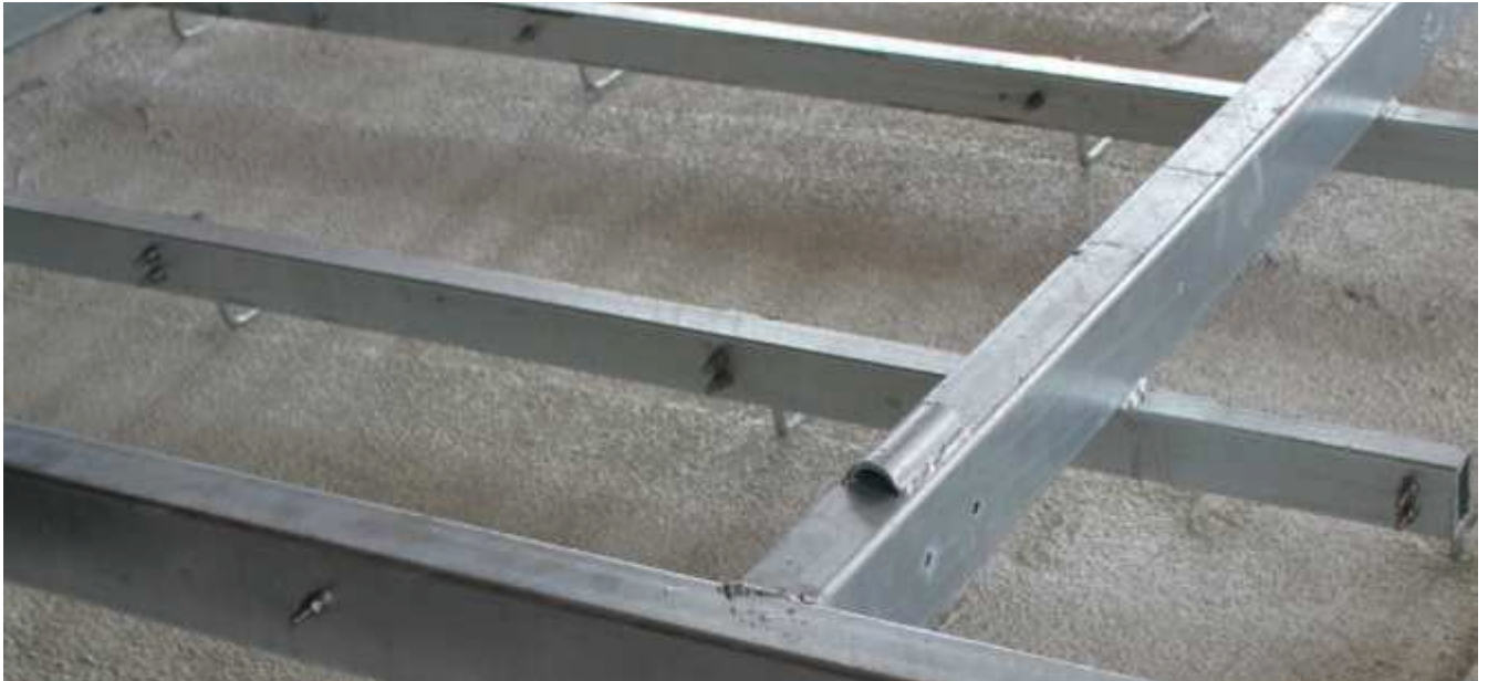
Figure 7 Connection of steel structure with the GRC panel backside
